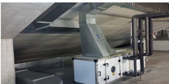
Figure 22: AP under-floor installation (not recommended)
