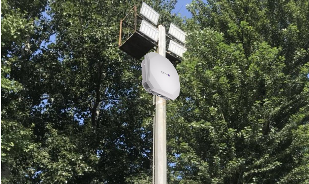
Figure 11: AP field area installation
