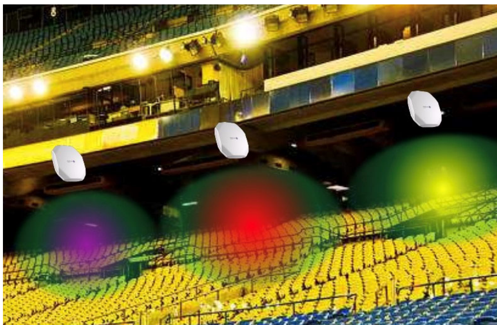
Figure 16: AP installation on the ceiling of the stadium
