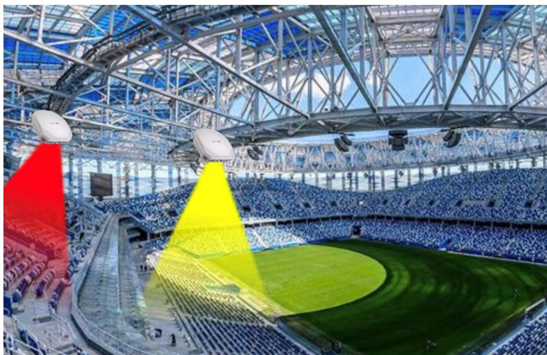
Figure 20: AP installation on the steel frames on the stadium roof
